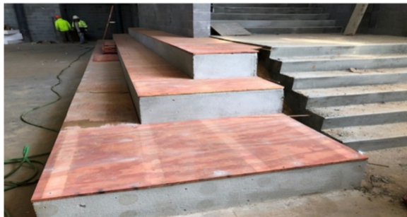
Installing wood at Bleachers at Gym
