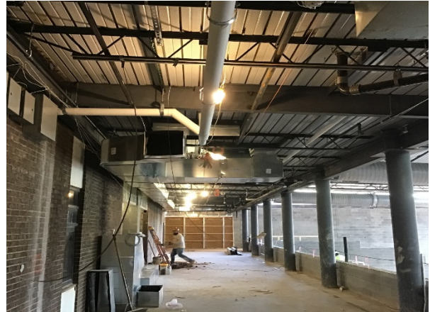
Hanging Ductwork at Overlook
